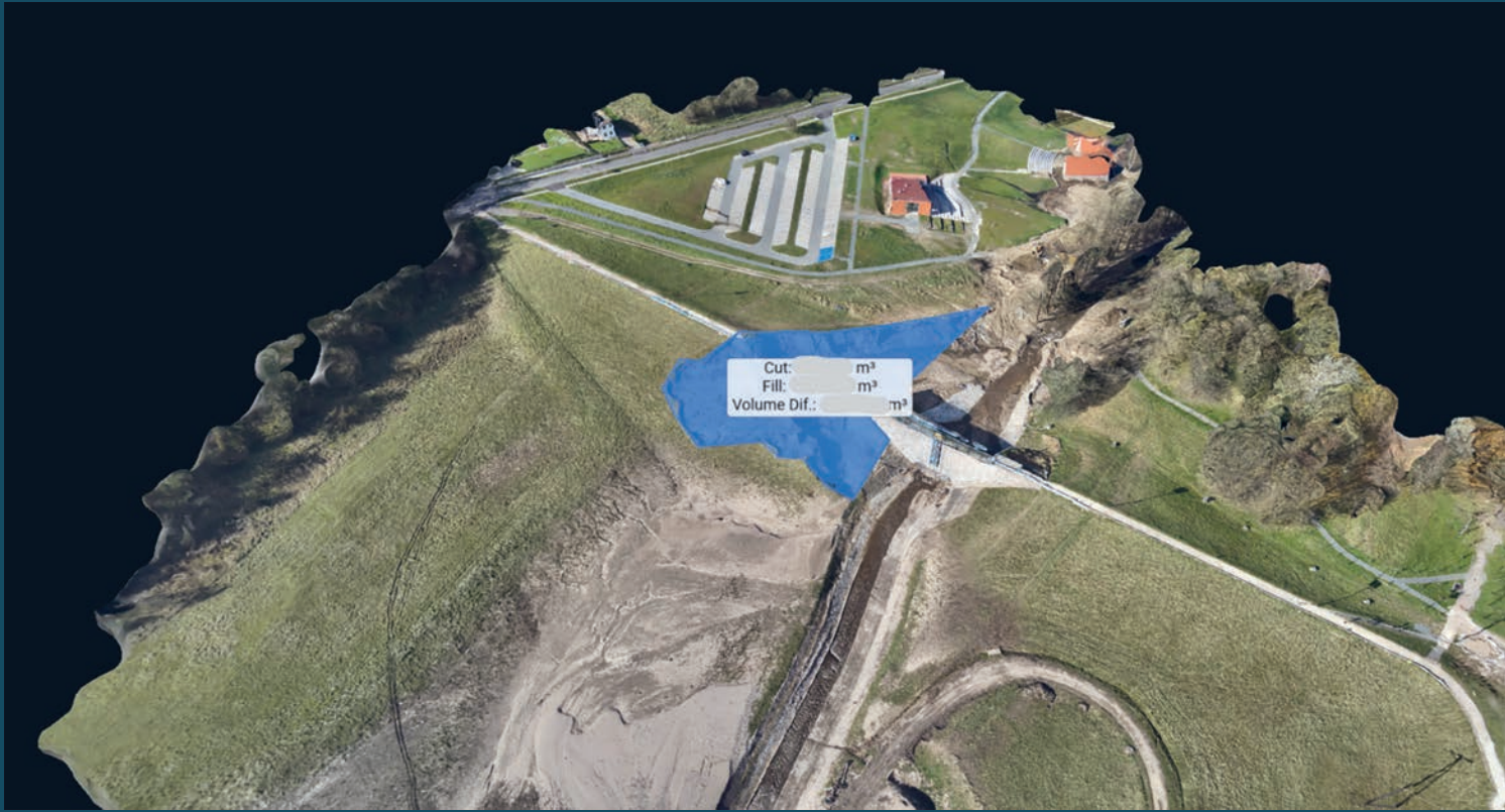
Dam on the Morawka River in the town of STRONIE ŚLĄSKIE. 8 min BSP DJI Mavic 3t raid with 8 ha coverage. Raid carried out to acquire a measurable 3D model to undertake a volume assessment the cavity created in the earth section of the dam embankment.
