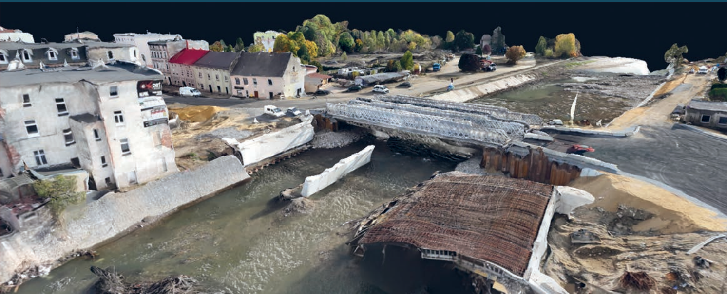
A model of the civil engineering structure, temporary bridge DMS - 65, built on the site of a destroyed bridge crossing. The cyclic raid of the BSP acquiring imagery for 3D modelling of the object allows for precise and continuous surveillance by the owner of the structure of its technical condition. At high rates implementation of a temporary structure in a post-flood area, it can be assumed that a selected part of the structure may be subject to unforeseen deformation. Dangerous deformations can be diagnosed by comparing several consecutive images.
